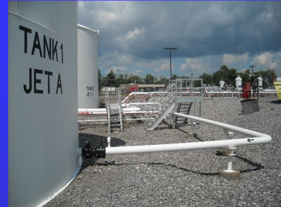
Tank Grounded to Other Structures
