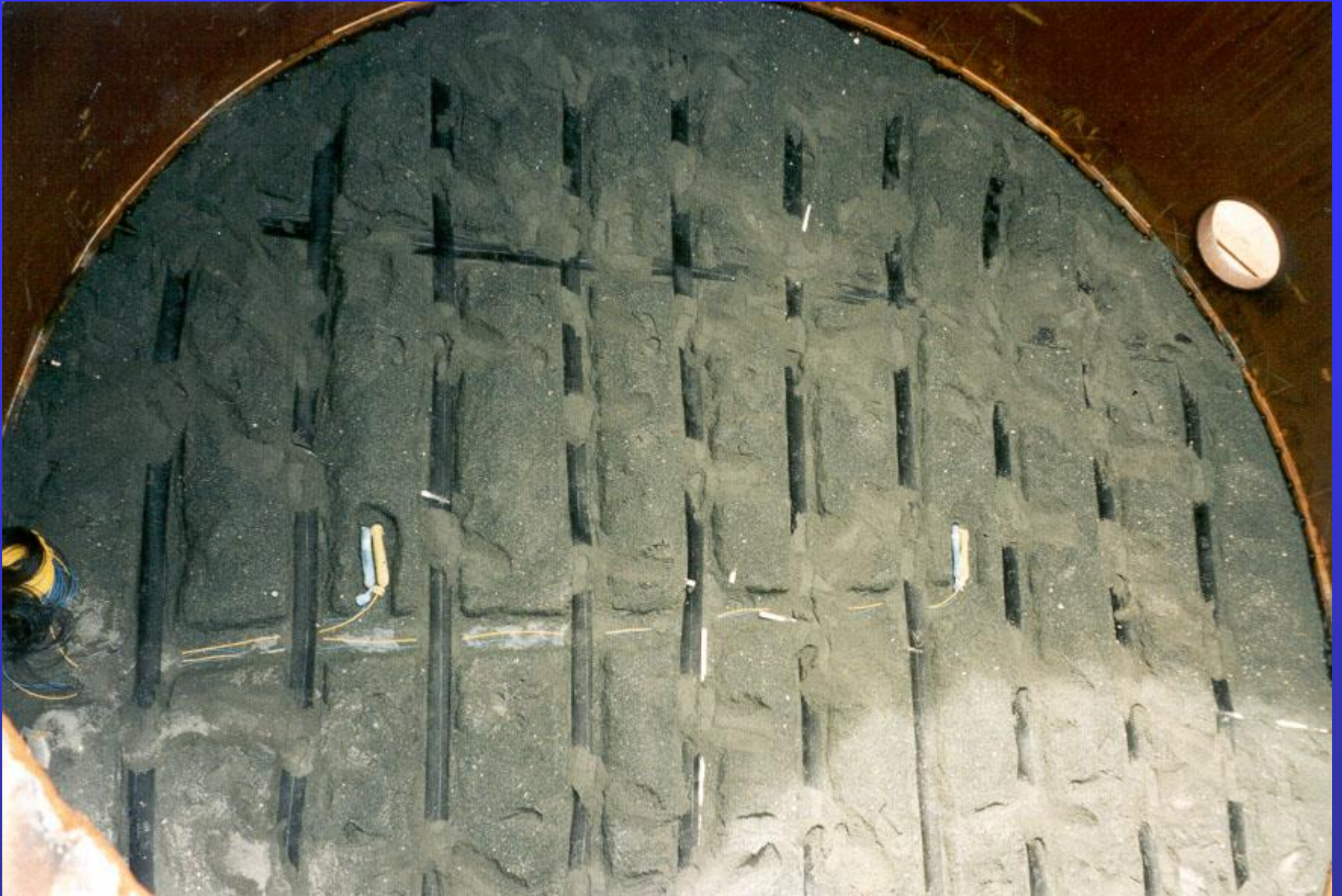
CP Installation on Rebottoned Tank
