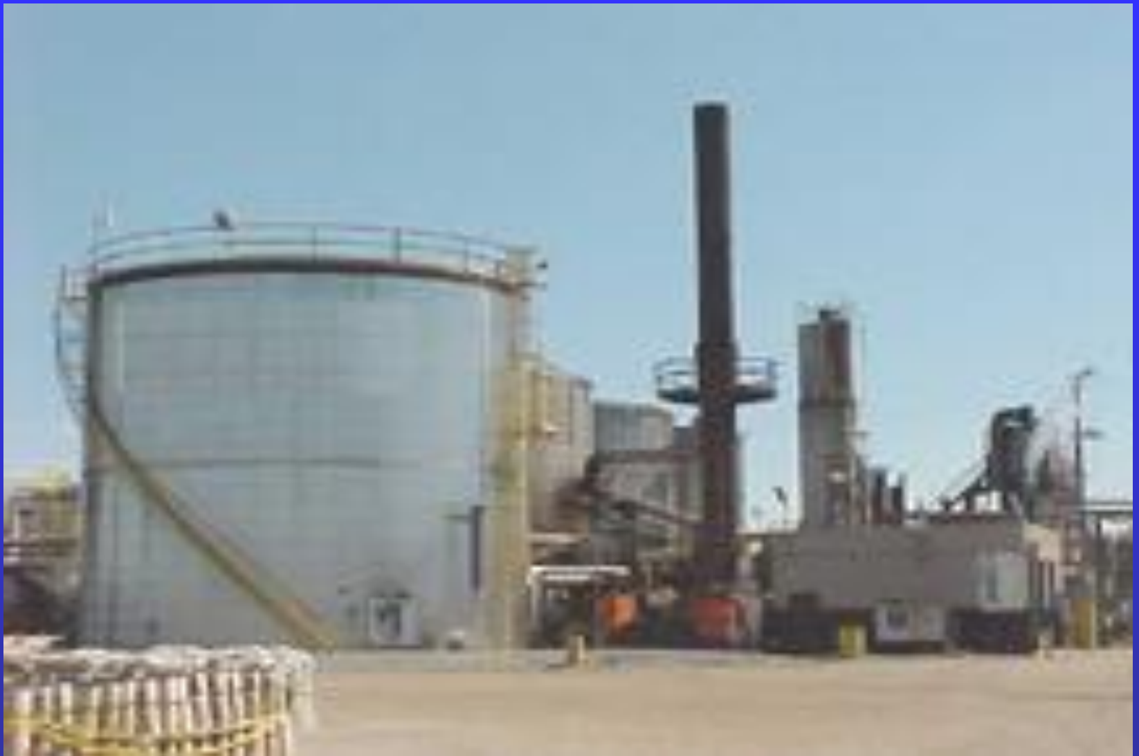
Hot Asphalt Tank Bottoms
