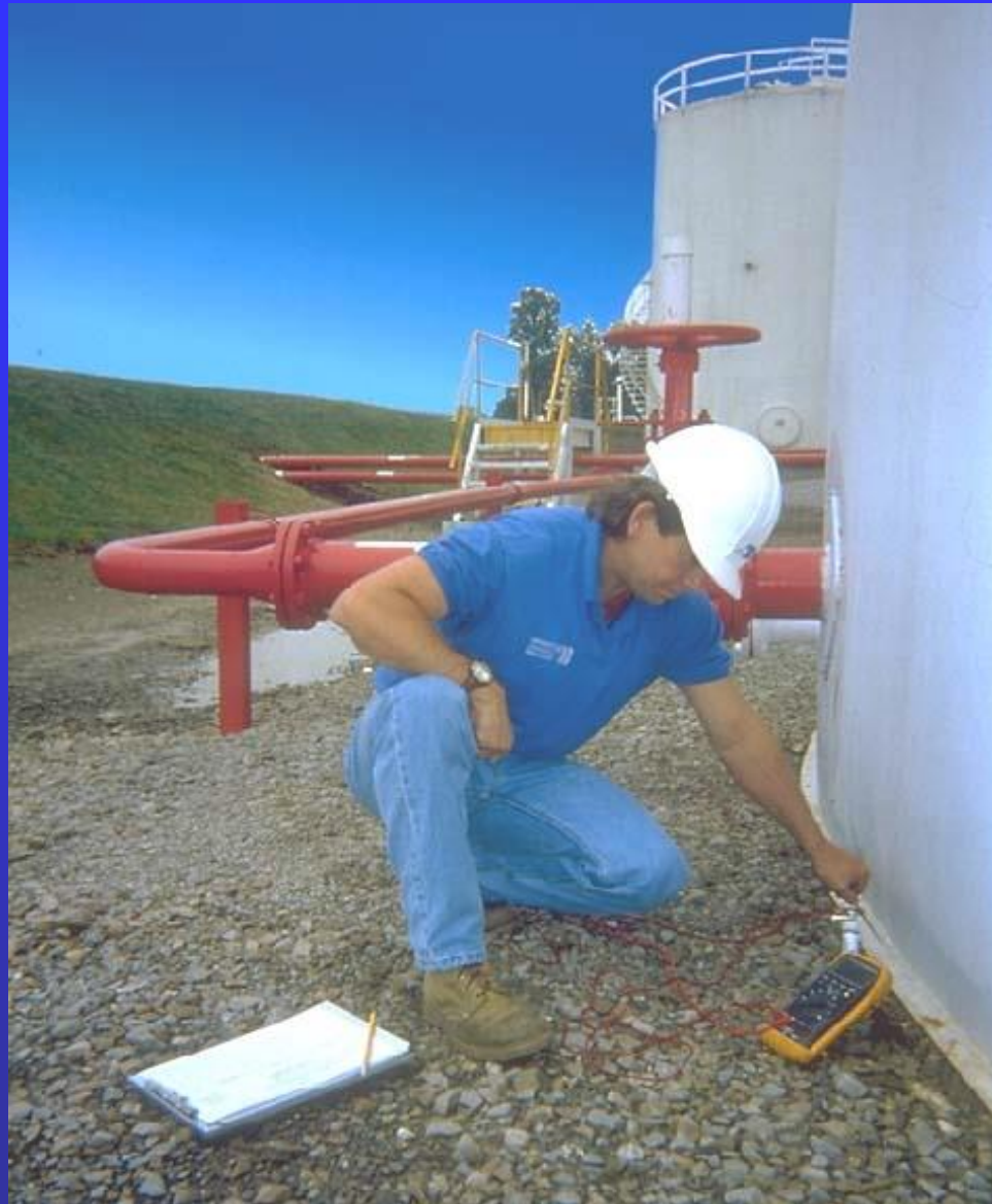
Cathodic Protection Survey (When Tank is Full)
