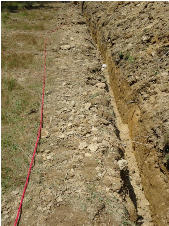
MULTIPLE INSTALLATION OF GALVANIC ANODES
