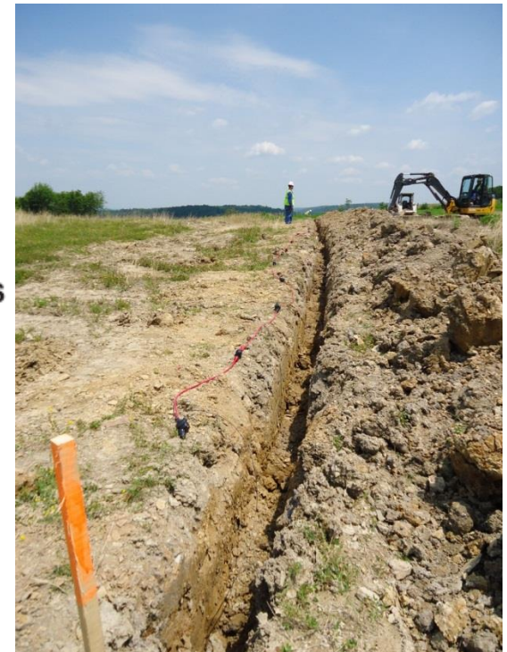
MULTIPLE INSTALLATION OF GALVANIC ANODES
