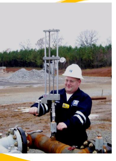
Injection atomizers, mixing probes and quills could require maintenance so retractable models should be considered.
