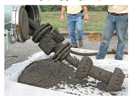
The most common method for cleaning pipelines relies on a device (pig) propelled through the pipeline pushing fluids and debris out.
