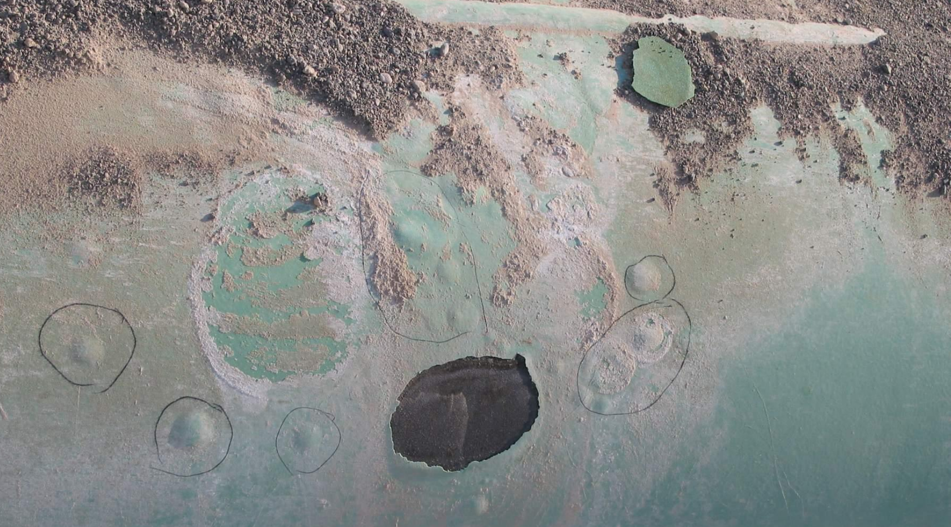
Close up of blisters on FBE coating and pipe under blisters. No corrosion.
