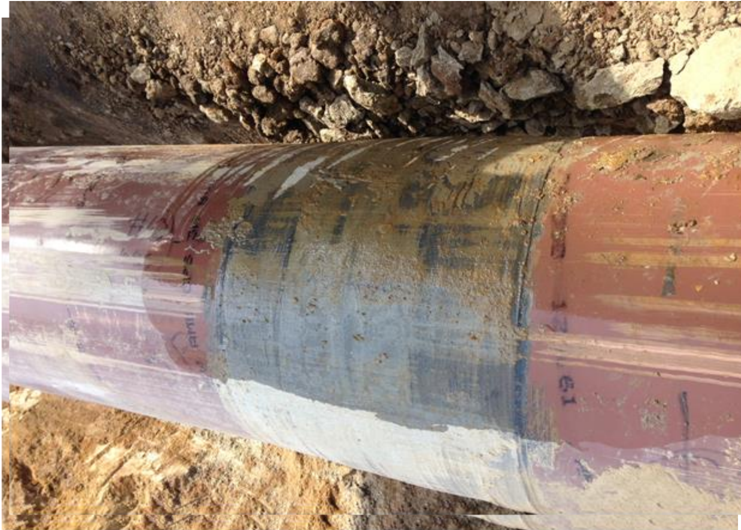
30" OD Pipe – shale conditions, damage to ML ARO
