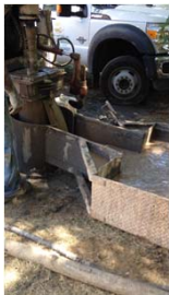
Drilling of anode well
