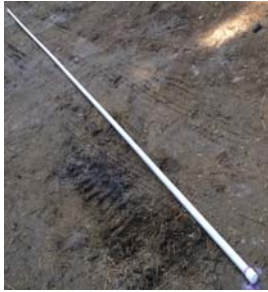
Installation of anode vent
