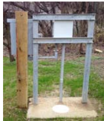
Completed installation of rectifier, anode junction box, and RMU. Anode well cap in pad.
