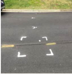
Paint markings showing crossing of WHC and gas main.
