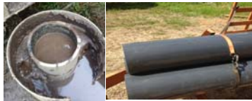
Anode well casing typically installed in first 50 ft of well
