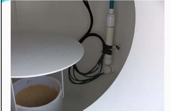
Fill pipe, pressure entrance fitting, and reference cell
