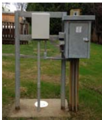
Completed installation of rectifier, anode junction box, and RMU. Anode well cap in pad.
