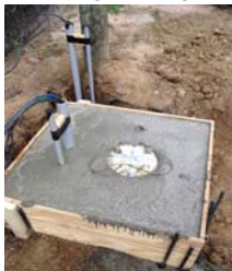
Anode well with vent cap attached, and anode leads in conduit for placement in junction box.
