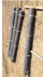
Centralizers attached holds anode in place in well.
