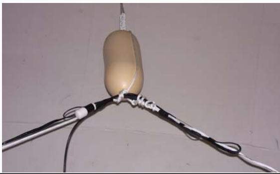
Feed wire connection to anode
