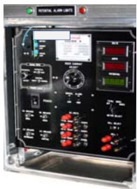
Potential Controlled Rectifier
