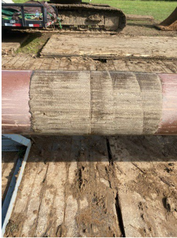
Figure 4-16: Outerwrap on Girth Weld After Pullback
