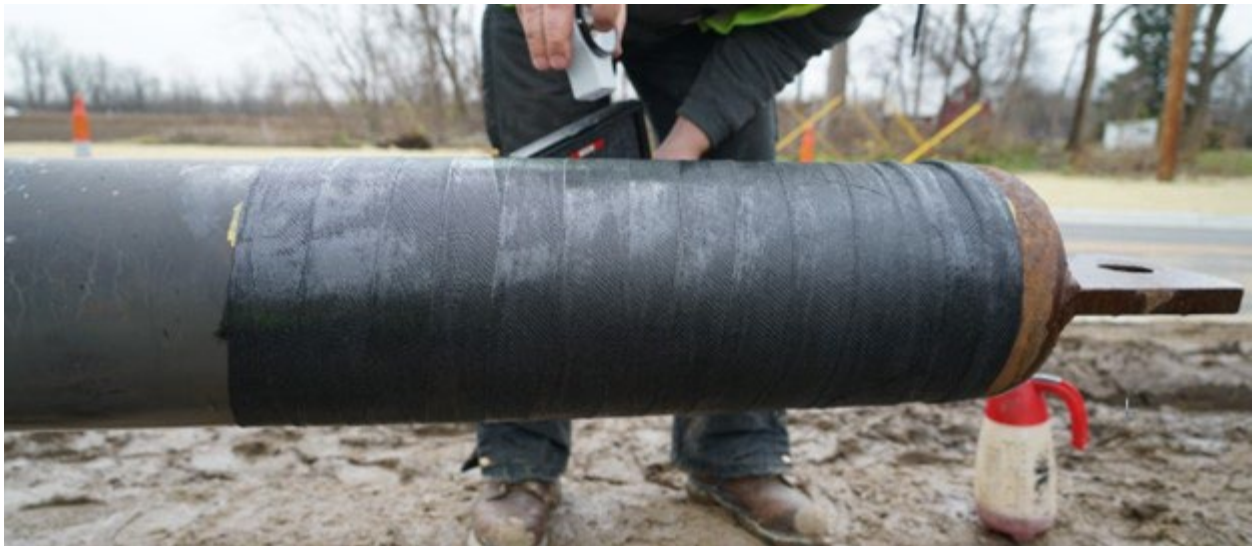
Figure 4-15: HDD Pull Head with Outerwrap Before Pulling
