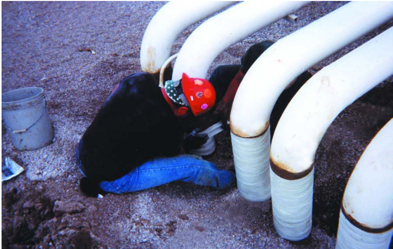
Figure 4-10: Applying Outerwrap Over Wax Tape
