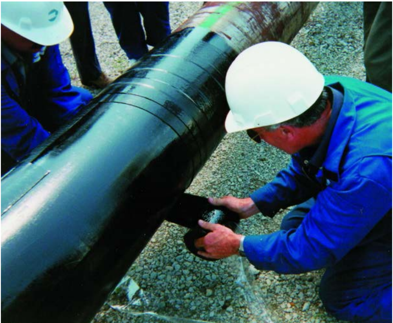
Figure 4-13: Cold Applied Tape
