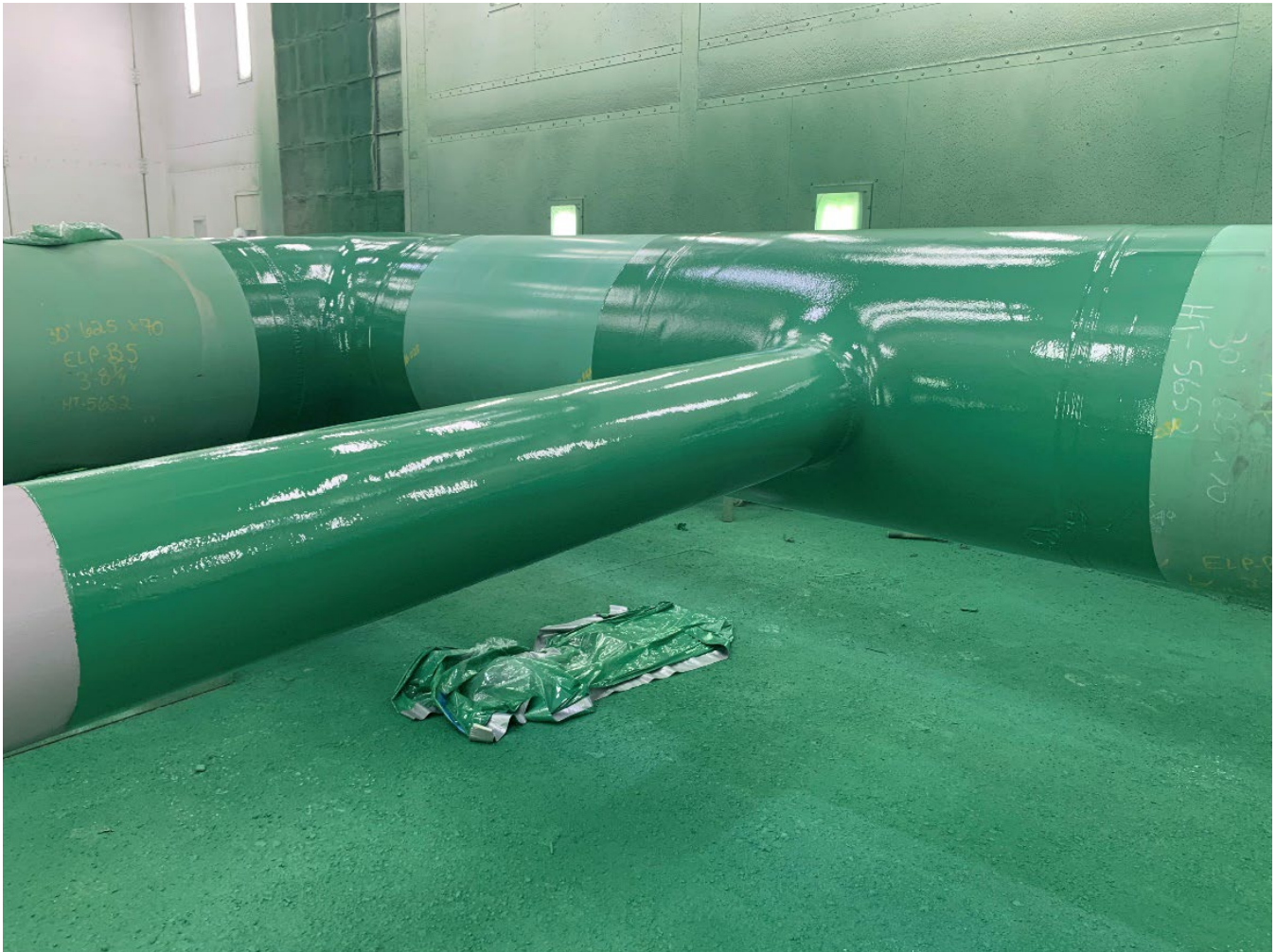
Figure 4-9: Plant Applied Liquid Epoxy
