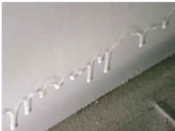
Figure 9-11: Runs, Sags, Curtains, Drips
