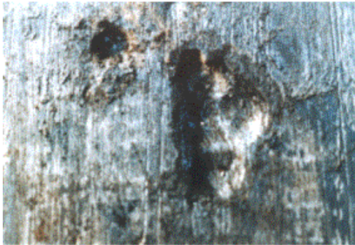
c. Pit products in b. removed
