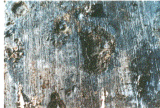
b. Corrosion in pit
