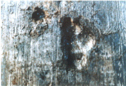
c. Pit products in b. removed
